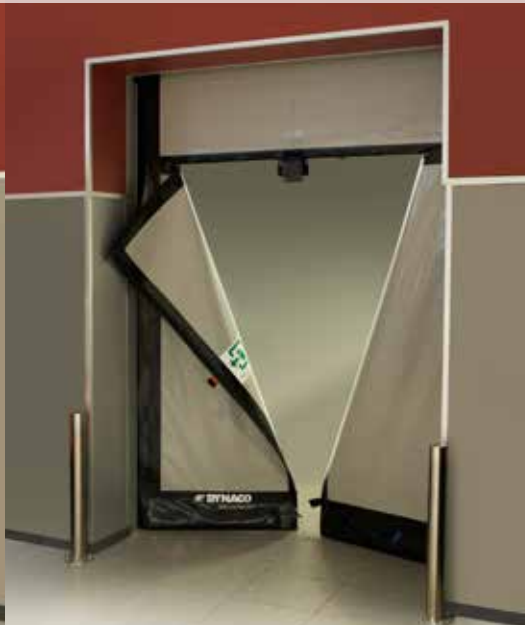
Emergency exit open
